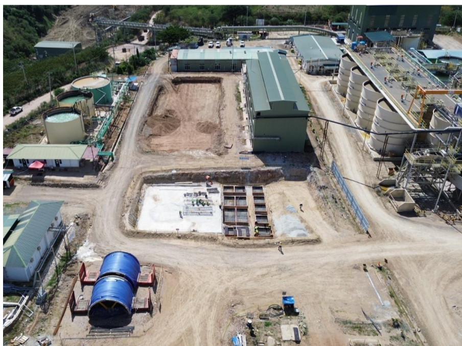
CPM CIL 1 Progress November 2025
