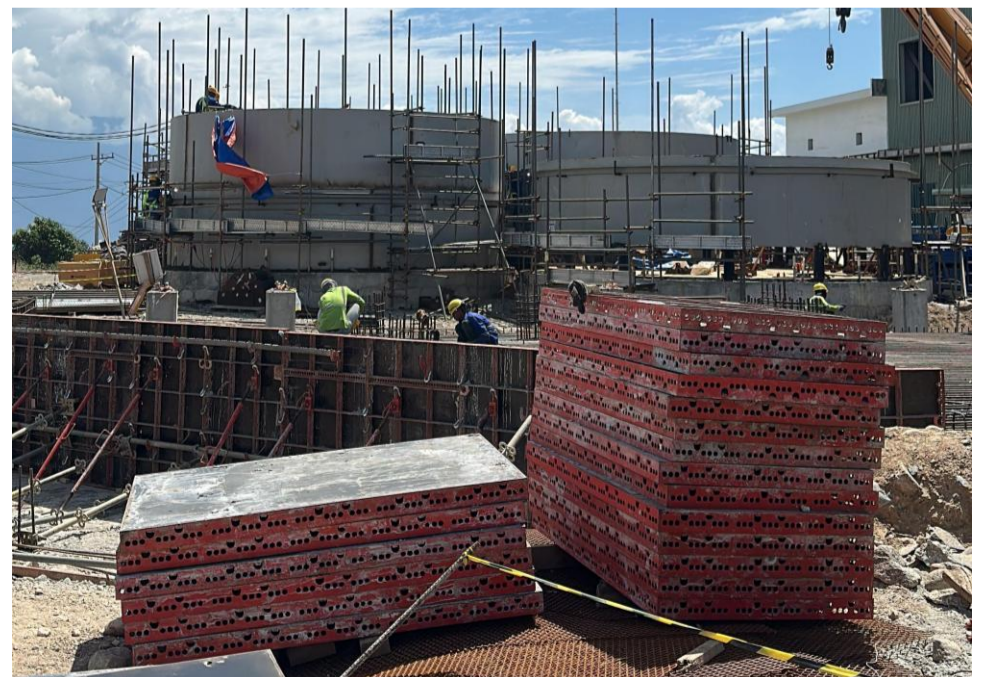
Figure 7. CIL Tank on CIL 1 Development Progress
